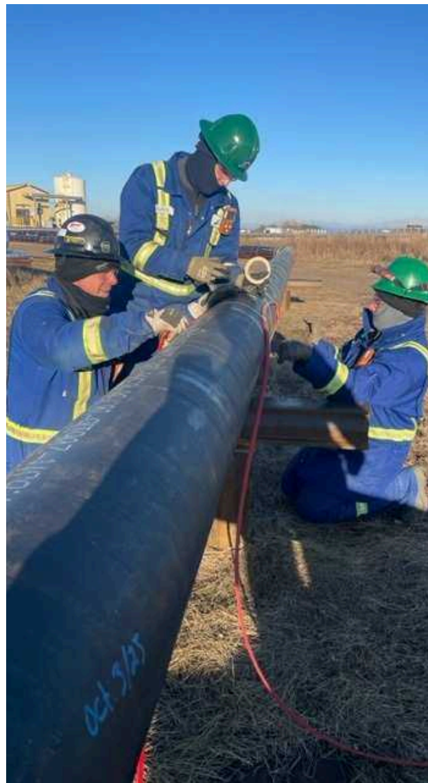
Pictured: A PTW journeyperson and two apprentices install electrical heat trace equipment on a new thermal production pipeline.
