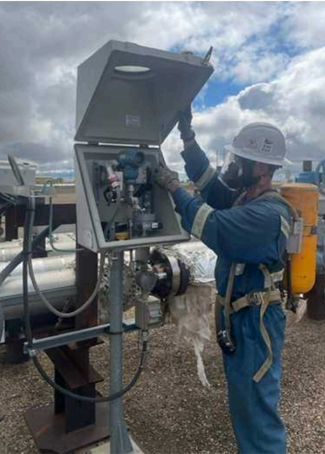
Pictured: A PTW worker is using SCBA supplied air while opening a sealed O'Brien box in a potentially high H2S environment.
