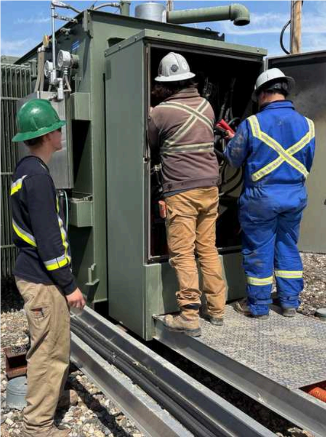
Pictured: Two journeyman electricians and one electrical apprentice remove connection hardware from a transformer.
